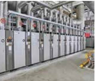
Gas-fired boilers installed at beer factory
