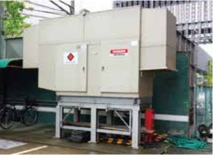
Backup power generator for head office functions
