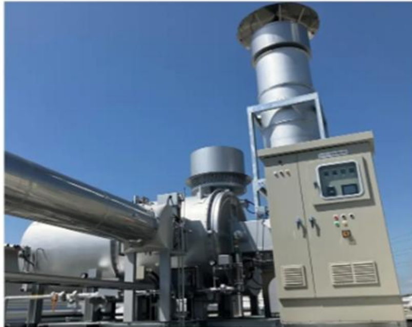
A testing facility for ship boilers equipped with ammonia dual-fuel burners, built on the premises of the MIURA Horie Plant in Matsuyama, Ehime Prefecture
