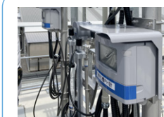
Installing water-quality meters
