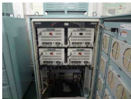
Inside of source panel (Source panel of door type)
