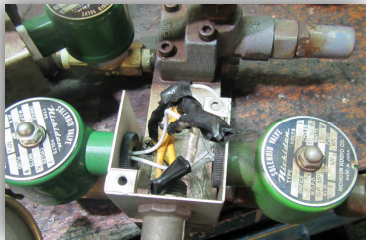
Wiring of solenoid valve for burner
