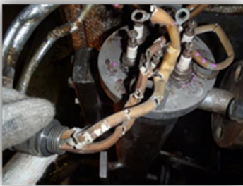
Wiring around water level gauge
