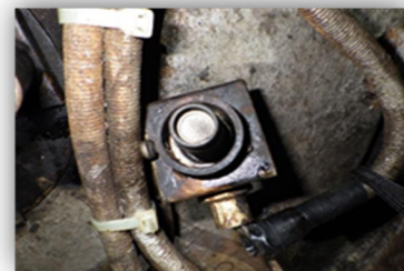
Wiring of flame eye
