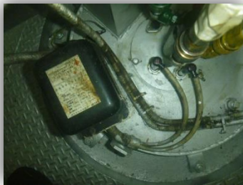
Wiring of ignition transformer
