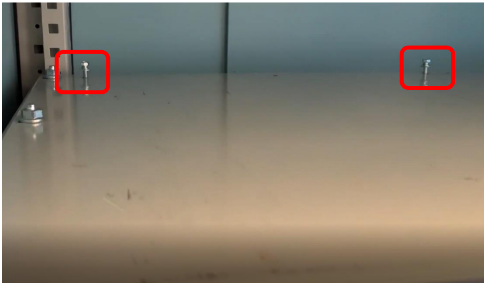
Figure 11 After installation of bolts with washers
