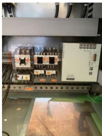
Figure 21 After installing switching power unit
