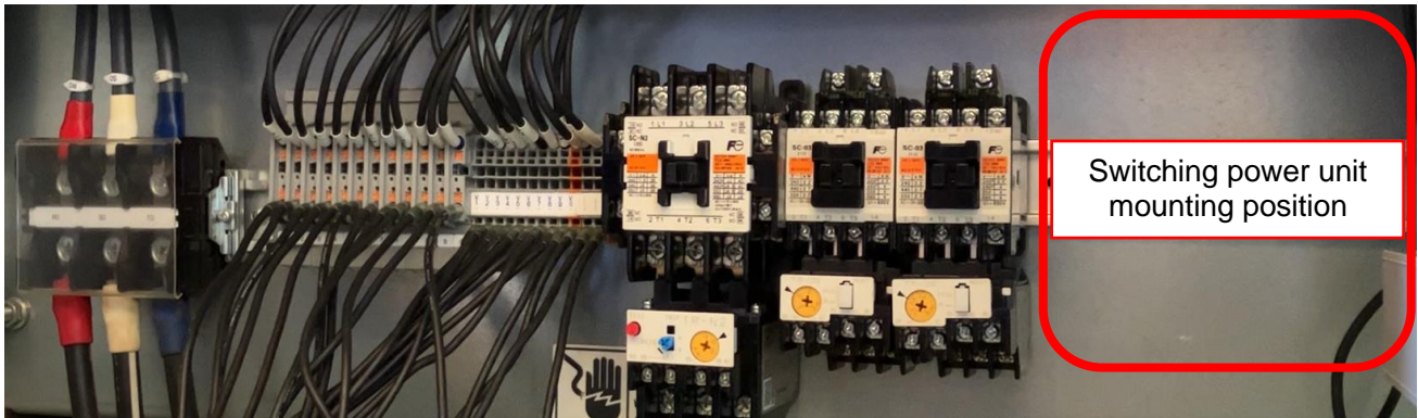
Figure 19 After attaching terminal block and contactor
