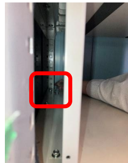
Figure 9 Removal of two bolts on the rear side
