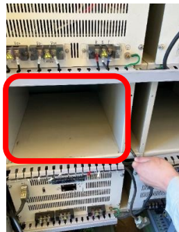
Figure 8 Space after pulling out 4 kW power unit
