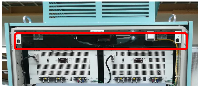
Figure 2 Acrylic plate on the top of the source panel
