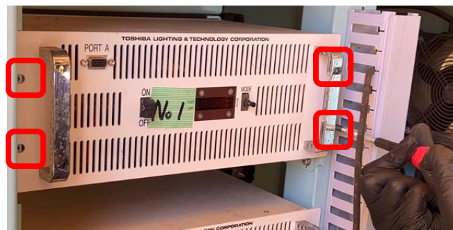
Figure 6 Removal of 4 kW power unit fixing screws
