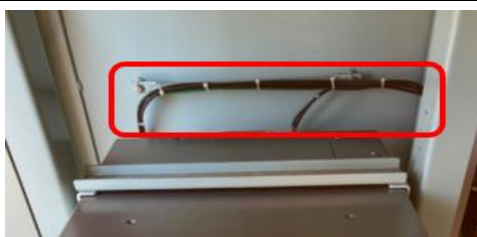
Figure 3 Wiring disconnection points on source panel side
